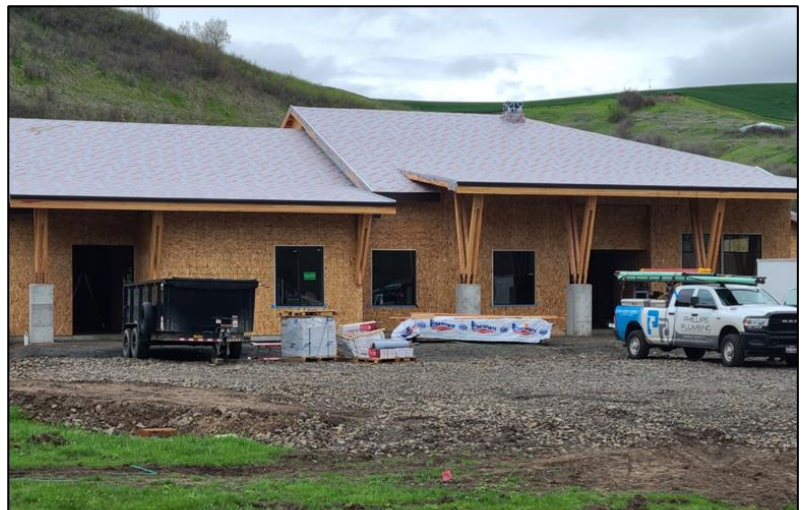
Assisted Living Facility Construction Progress
